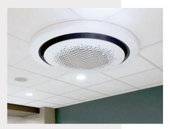
Plasma Air model PA664 was installed in multiple VRF round cassettes and ducted air handling units.
